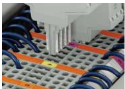
Coding ensures correct polarity.
