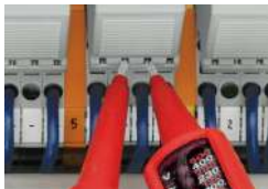
Function testing via touch-proof test slots
